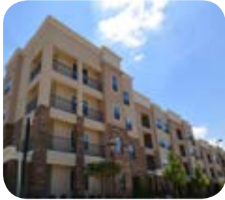
Terraces at Suwanee Gateway Suwanee, GA Units: 335
